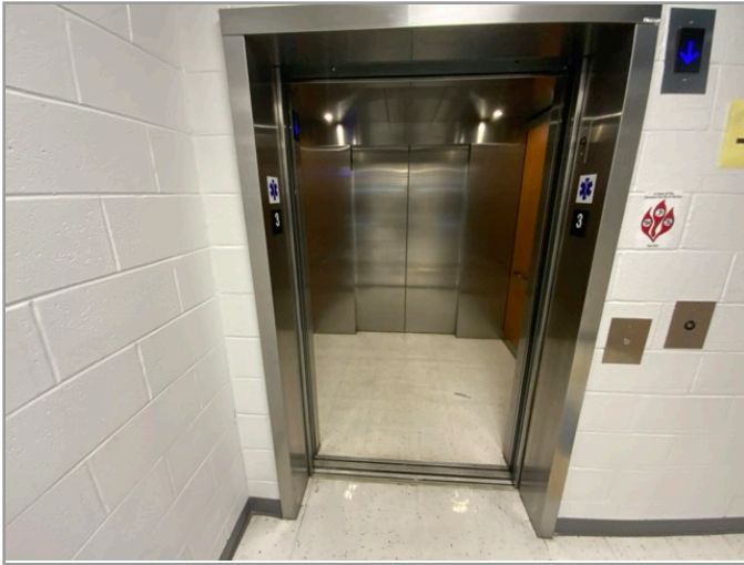
LOBBY LOOKING AT CABS
