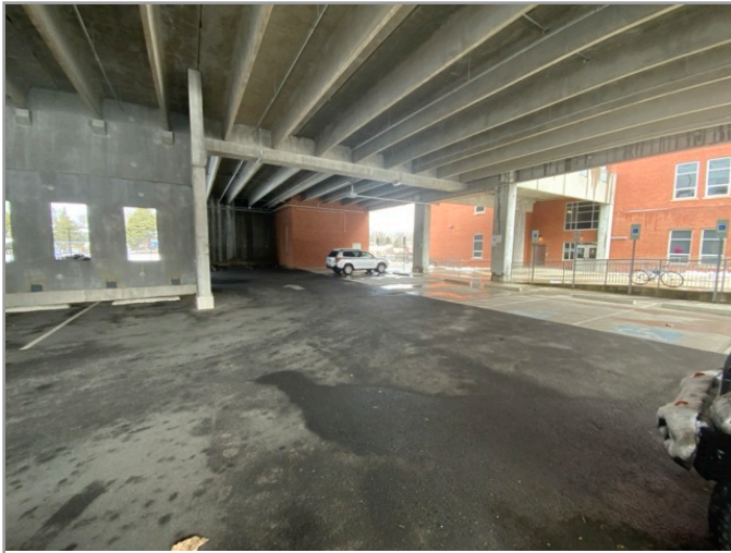
OVERVIEW OF ACCESSIBLE PARKING AREA
